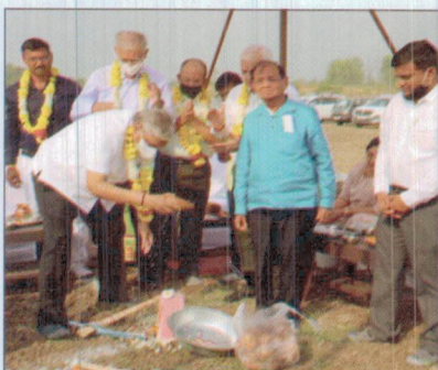
President Shri Bharatbhai laying foundation stone at Amalsadi
