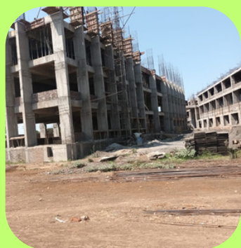
Amalsadi construction progress
