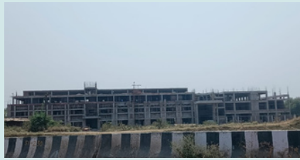
Amalsadi constructions progress
